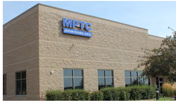
The new Jackson Regional Center.
